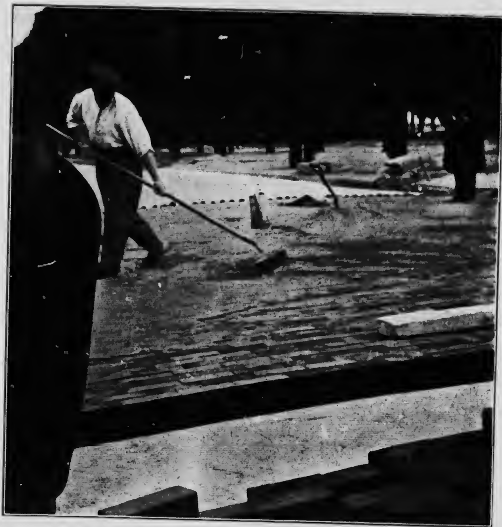
Photo by permission of Mr. S. R. Church, Barrett Mfg. Co., New York. Laying 5-inch deep Swedish pine wood block in Paris. Cours la Reine—Applying cement-sand grout to the surface of the pavement.
