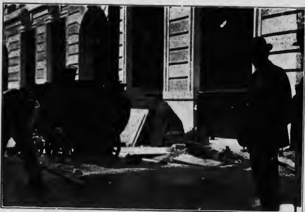
Laying 5-inch creosoted deal blocks on concrete foundation, Gracechurch street, London. Squeegging the pitch flush coat.
