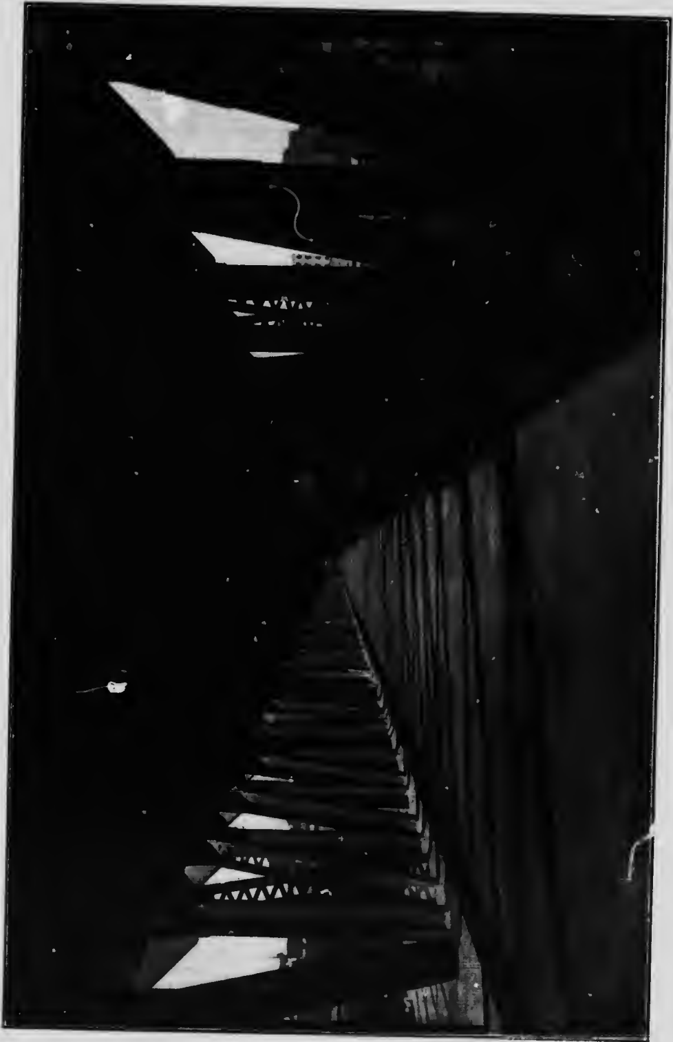
C. P. R. High Level Bridge, Edmonton. Highway floor paved with creosoted wood blocks. By permission of Canadian Wood Preserving Co., Winnipeg.
