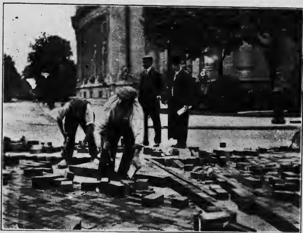
Photos by permission of Mr. S. R. Church, Barrett Mfg. Co., New York. Laying 5-inch deep Swedish pine wood block in Paris. Cours la Reine—illustrating the expansion joint.
