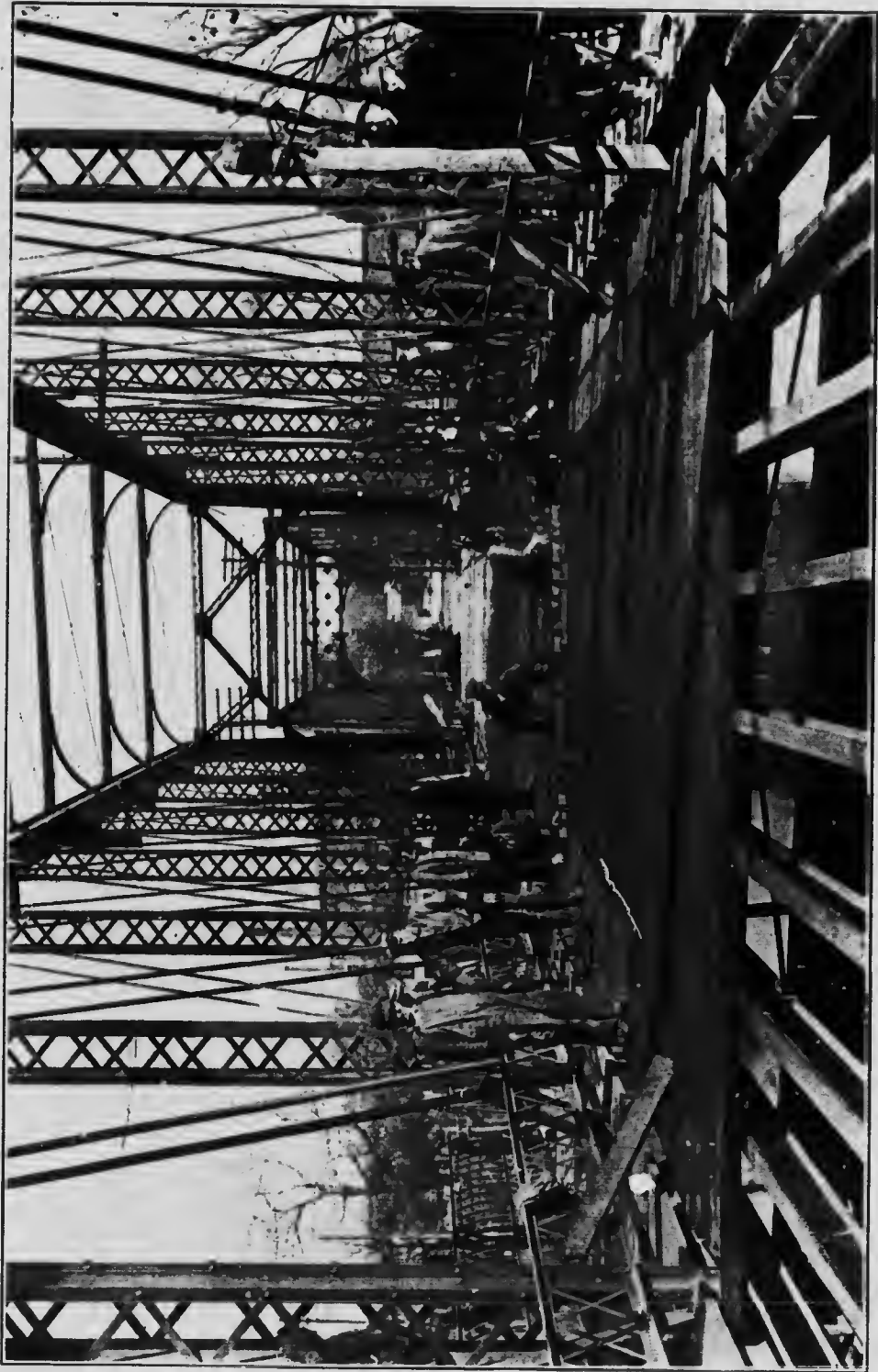
Construction of Creosoted wood-block pavement on highway bridge, Piqua, Ohio. By permission of Republic Creosoting Co., Indianapolis.
