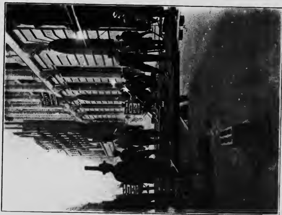
Photos by permission of Mr. S. R. Church, Barrett Mfg Co. New York. Laying 5-inch cross-acted deal blocks on concrete foundation, Gracechurch street, London. General view of the work.
