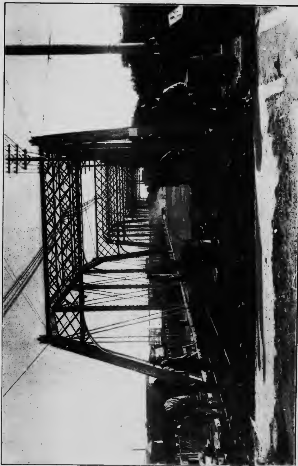
Main St. Bridge, Winnipeg—Paved with Creosoted Wood Paving Blocks. By permission of Canadian Wood Preserving Co., Winnipeg.
