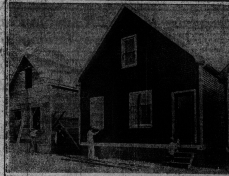
This shows one cottage being finished and one in course of construction. These cottages are well constructed—Manitoba siding, tar paper lining, heavy side boarding, and plastered. Only $1,200—and you will wonder how we did it for the price when you see them.
