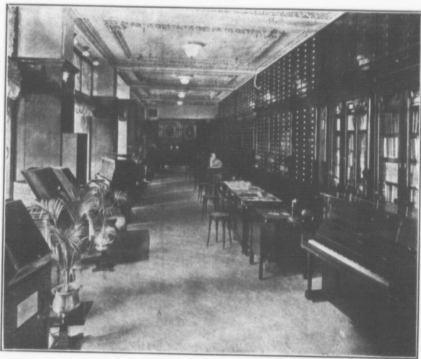
View of the ground floor at Nordheimer's, from the main entrance.
