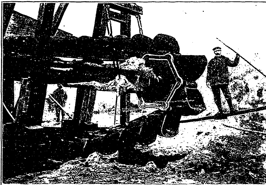
Buckets of the Robinson Gold Mining Dredge.
