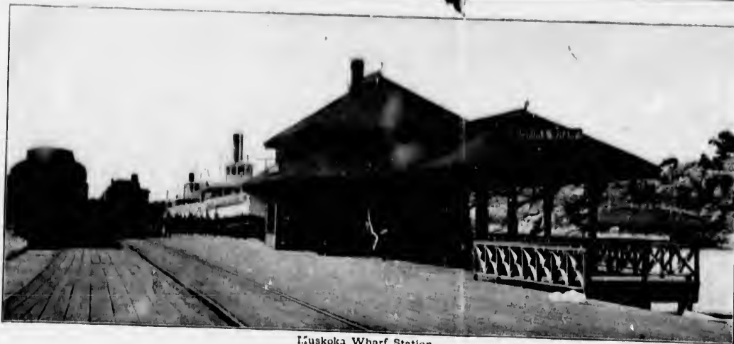
Muskoka Wharf Station.
