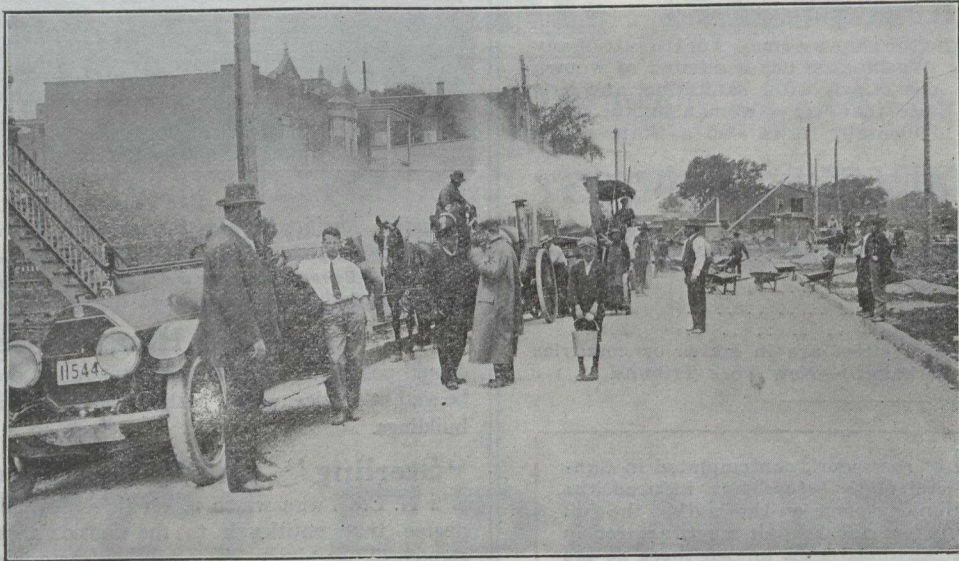
Constructing Penetration Road with Standard Asphalt Macadam Binder "B" Ville St. Pierre, near Montreal, Que.
