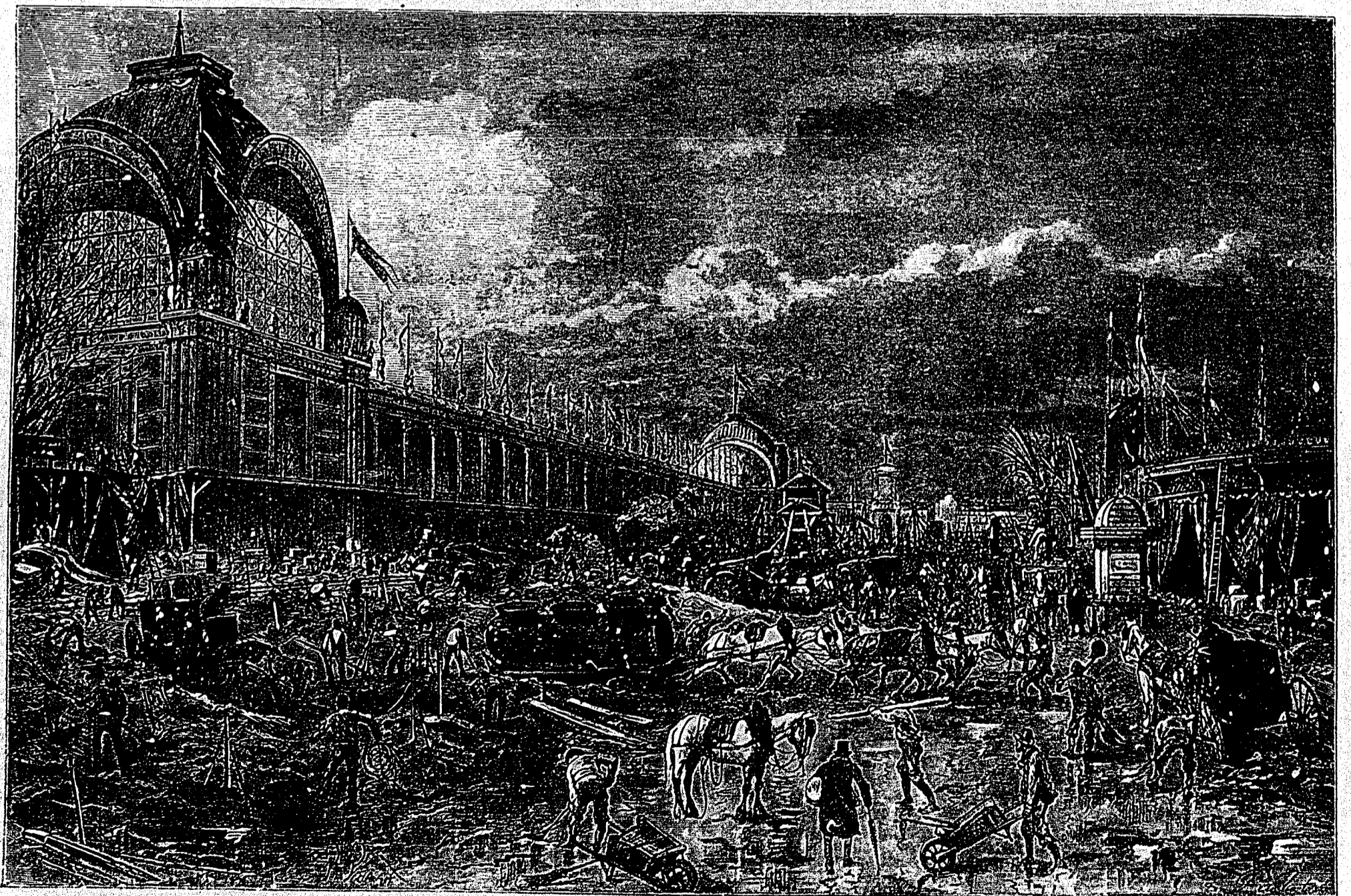
REMOVING GOODS FROM THE PARIS EXHIBITION BUILDING, PRIOR TO DEMOLITION.
