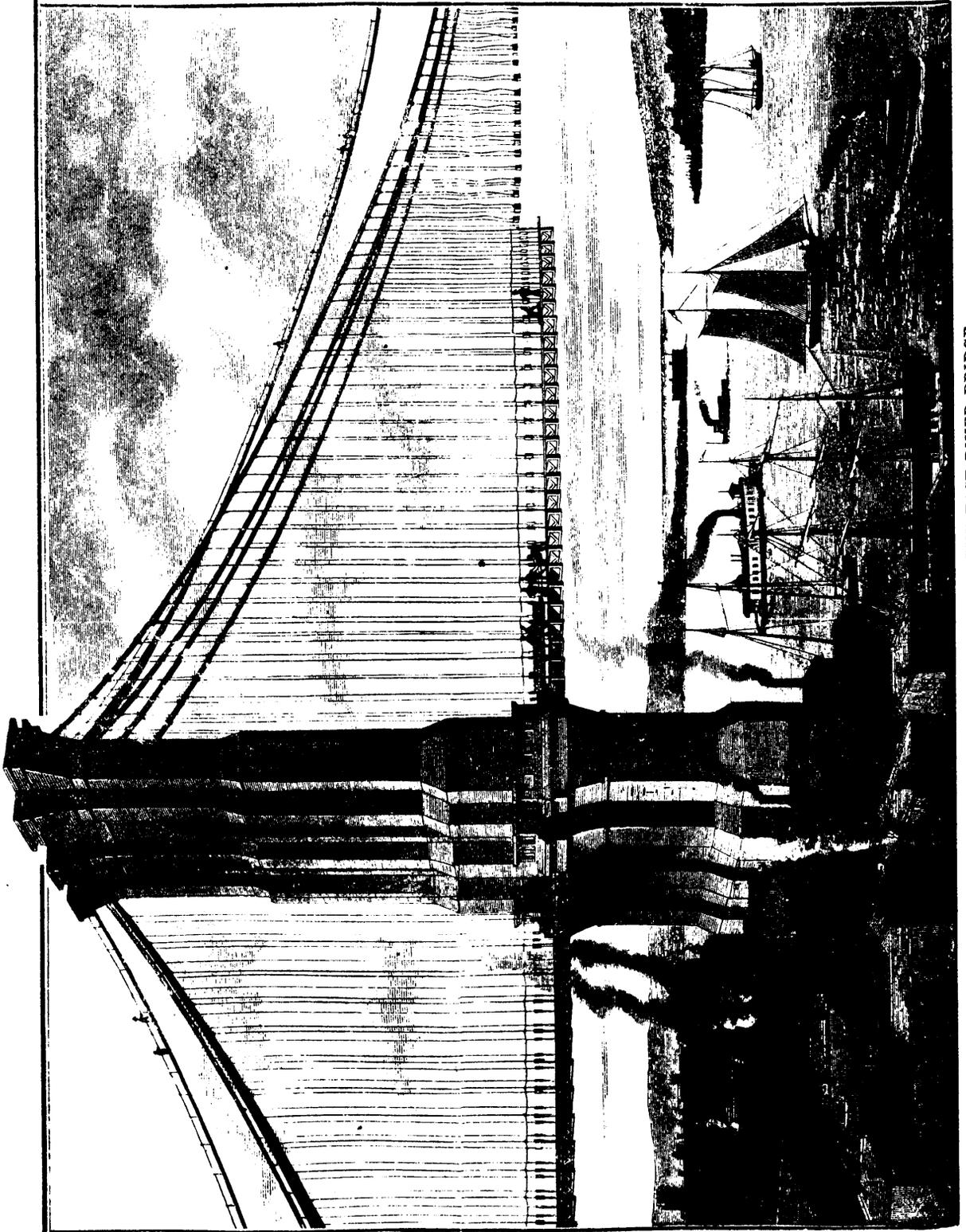
SUSPENDING THE FLOOR BEAMS OF THE EAST RIVER BRIDGE.
