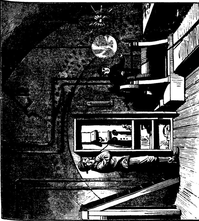
FIG. 4. TELEPHONE AND WINDLASS IN CAISSON.
