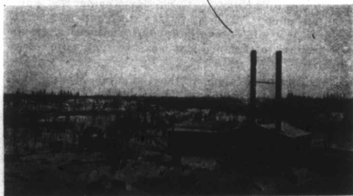
Power House and Shaft, Brooklyn Mine.
