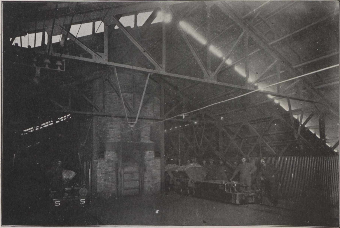
Blast Furnace Charging Floor, Copper Cliff Smelter
