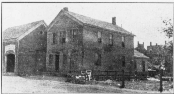
A DILAPIDATED DWELLING BADLY OVERCROWDED.
