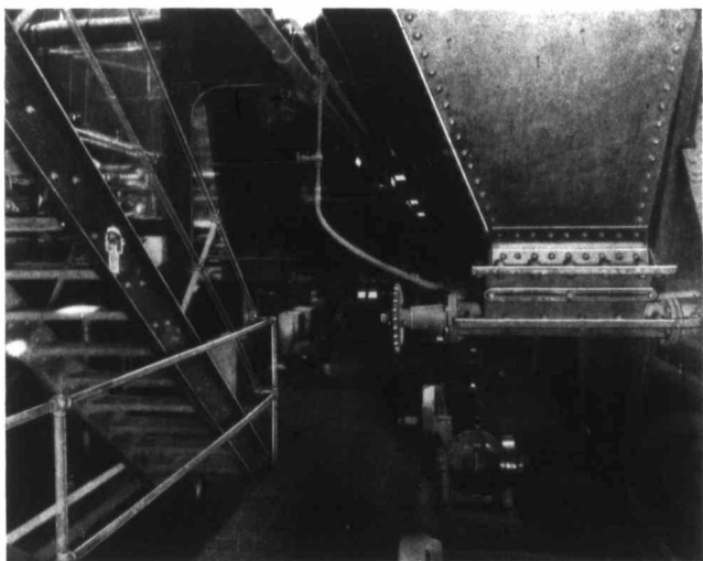
BRITISH COLUMBIA SUGAR REFINING CO., VANCOUVER, B.C. Pulverized coal equipment, on Badenhausen boilers, installed by Fuller Engineering Company.
