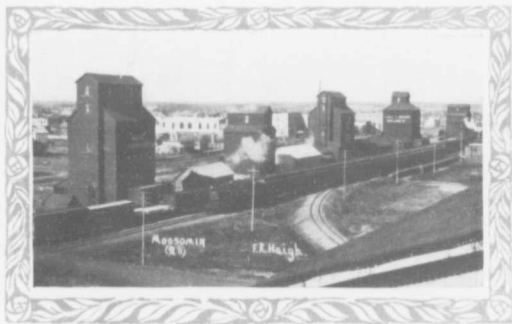
Elevators at Moosomin.
