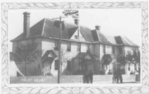
Court House, Moosomin.
