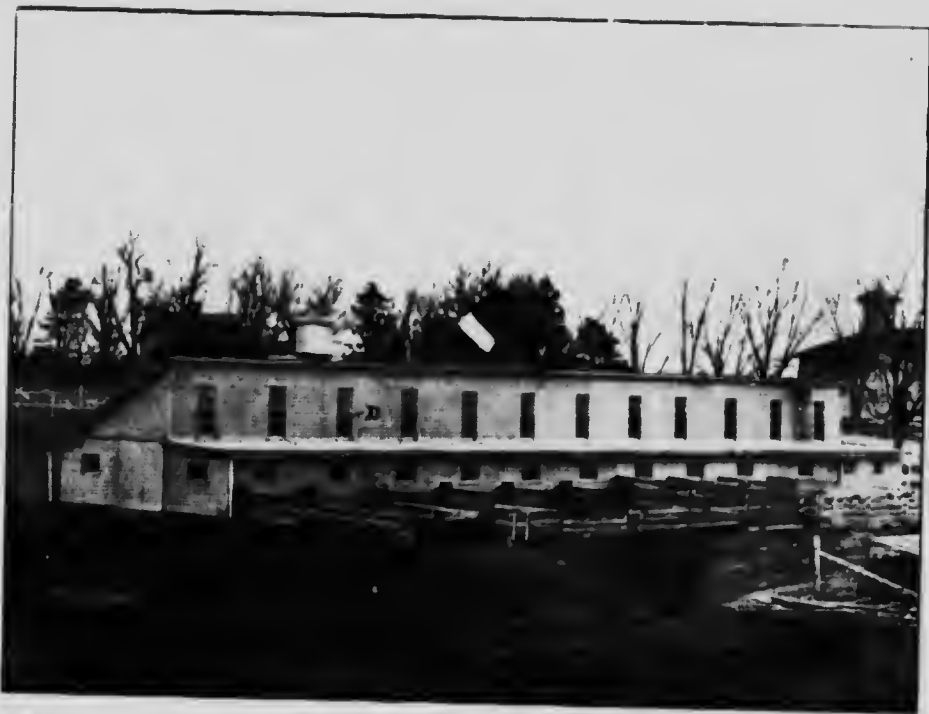
Fig. 27. A well lighted Piggery. Lower windows light the south row and upper windows the north row of pens.
