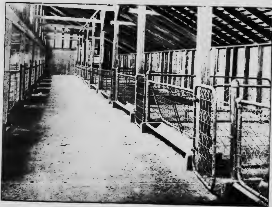
Fig. 28.—Interior view of well lighted Piggery showing the north row of pens lighted from the upper windows.
