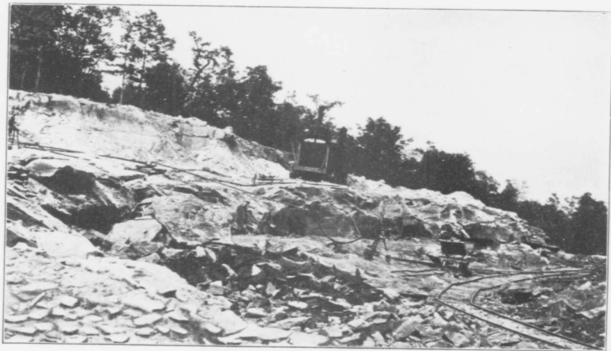
Typical quarry of bituminous sand-rock, operated by Wadsworth Stone & Paving Co., at Asphalt, Ky., U.S.A. Average thickness of bituminous rock 12 to 14 feet. Overburden consists of earth, loose rock and sandstone of average thickness of 10 feet.
