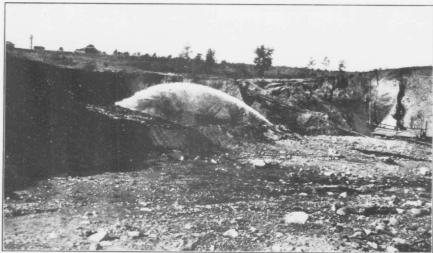
Rowe mine, Minnesota. General view illustrating hydraulic removal of overburden and showing water supply pipe, discharge pipe, and hydraulic gun.
