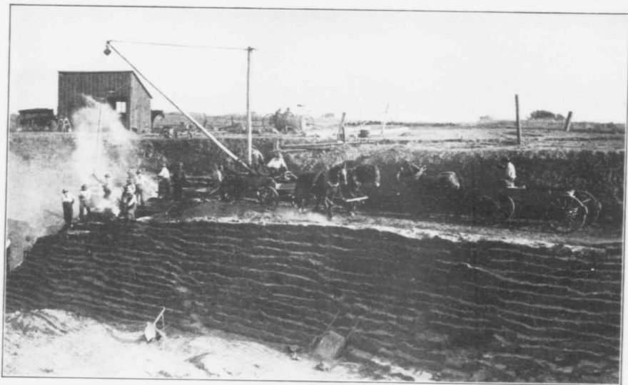
Quarry of soft bituminous sand near Carpinteria, Cal., U.S.A. The bituminous sand is 10 to 15 feet in thickness, overlaid by 8 to 10 feet of earth. The bituminous sand is excavated in a series of steps, heated spades being used in this work.
