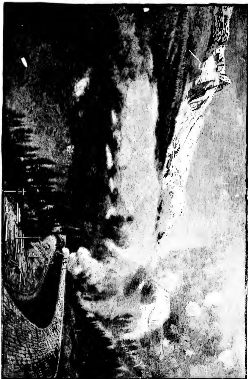
SNOW-SHEDS, SELKINK MOUNTAINS, THE WINTER TRACK UNDER COVER: THE OUTER TRACK FOR SUMMER USE.
