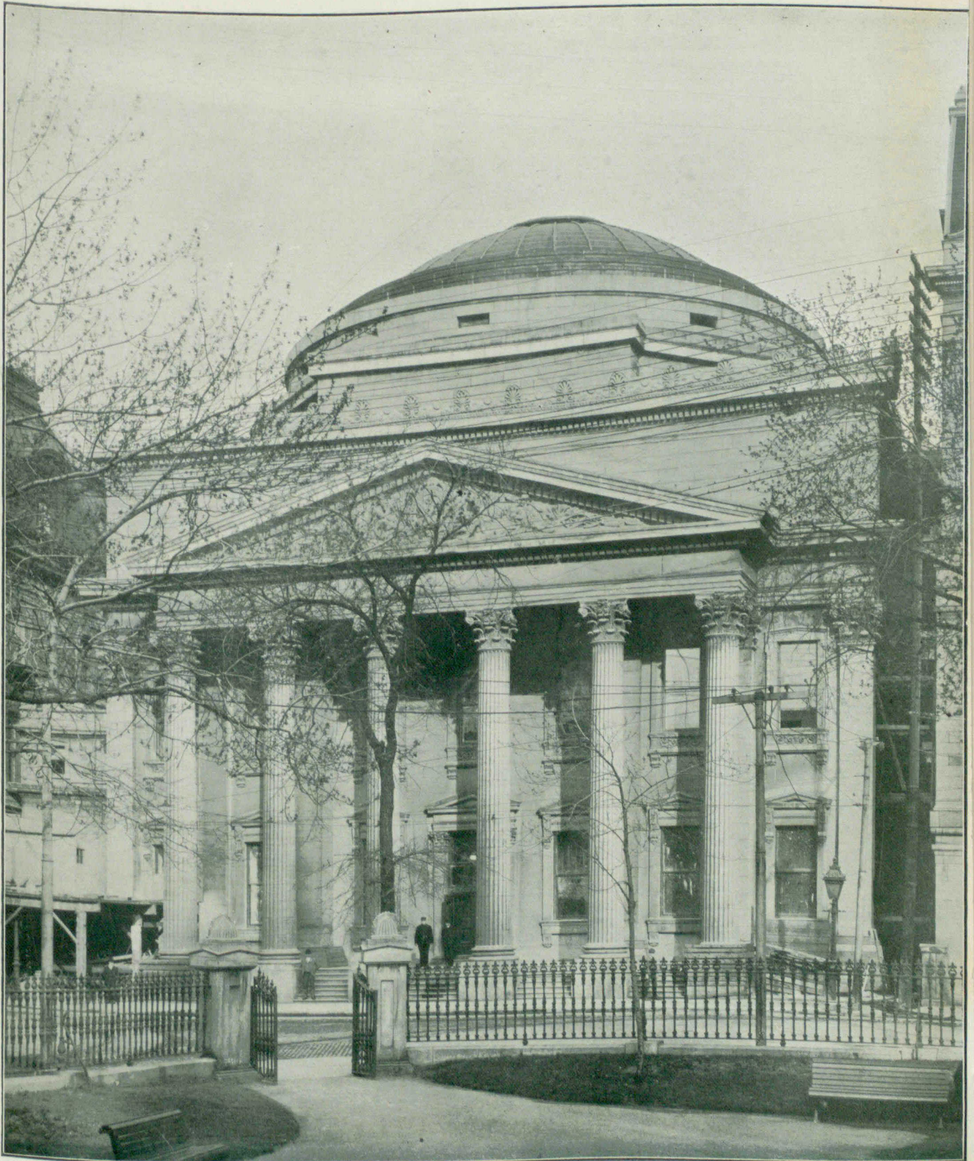
HEAD OFFICES OF THE BANK OF MONTREAL, MONTREAL, RECENTLY REMODELLED. MCKIM, MEAD & WHITE AND TAYLOR, HOGLE & DAVIS, ASSOCIATE ARCHITECTS.
