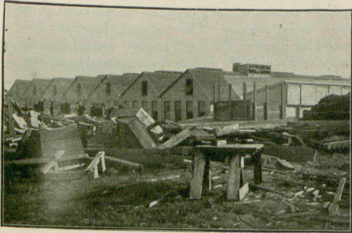
FIG. 2.—EXTERIOR VIEW OF FOUNDRY, SHOWING "SAW-TOOTH" ROOF CONSTRUCTION.
