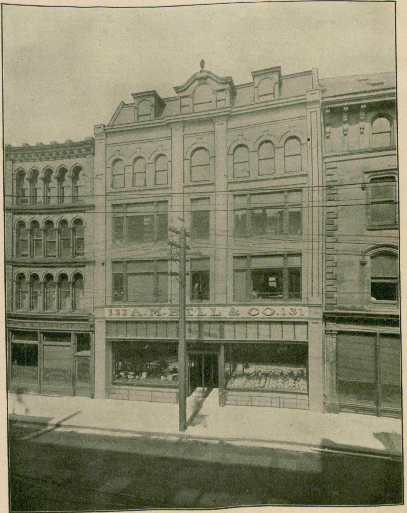
STORE BUILDING, HALIFAX, NOVA SCOTIA.
