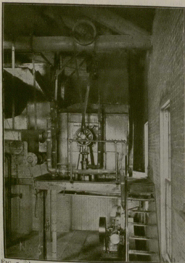
FIG. 7.—INDUCED DRAFT FANS, SHOWING STOKER ENGINE BELOW PLATFORM, AND PORTION OF GREEN FUEL ECONOMIZER AT LEFT HAND.
