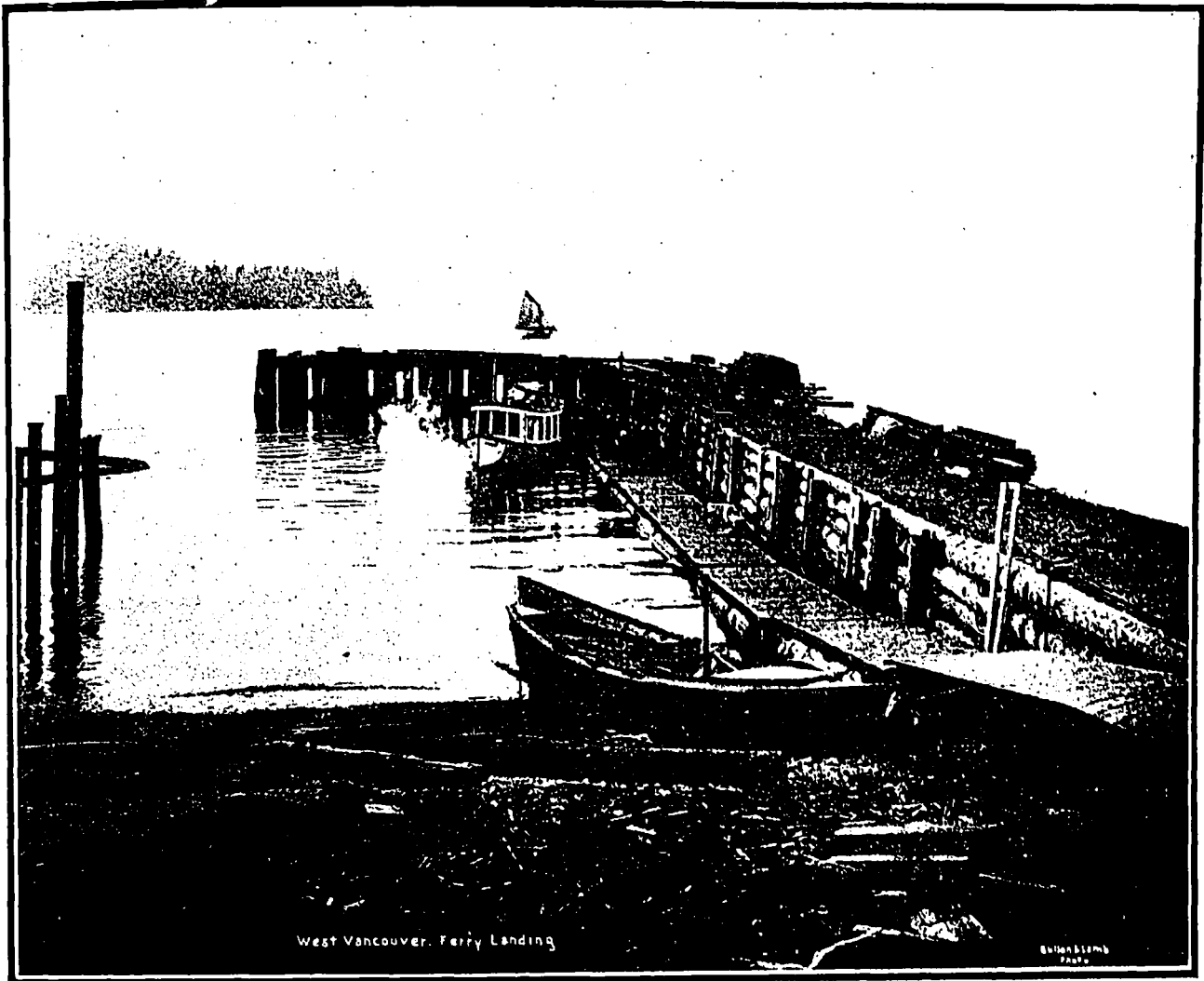
THE PRESENT CRIB WHARF AT HOLLYBURN. CONCRETE WHARVES WILL SHORTLY BE BUILT AT THIS POINT AND DUNDRAVE, WHICH IS FARTHER WEST
