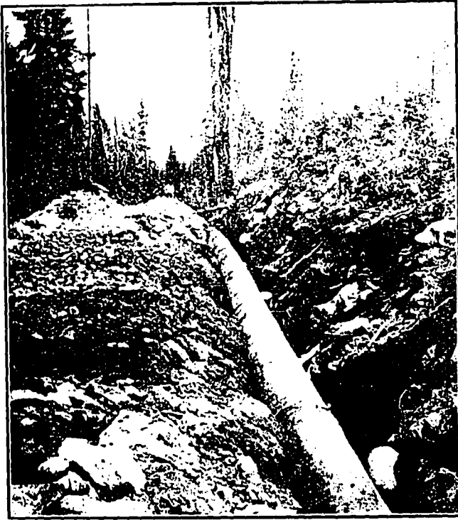
24-INCH LAP-WELDED STEEL MAIN, SEYMOUR CREEK
