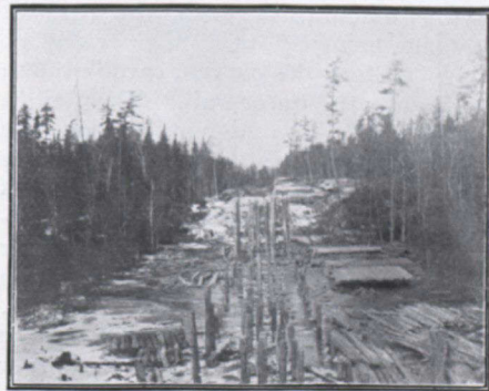
PILES FOR TRESTLE WORK
