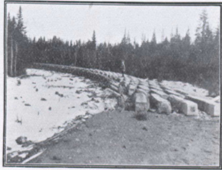
THE BEGINNING OF THE TRESTLE WORK
