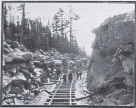
THE CUTTING COMPLETED AND THE RAILS LAID, AWAITING THE BALLAST
