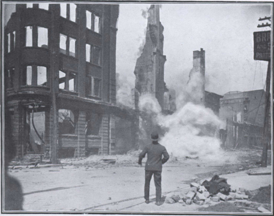
DYNAMITING THE DANGEROUS WALLS AFTER THE FIRE—PHOTO TAKEN AT INSTANT OF THE EXPLOSION
