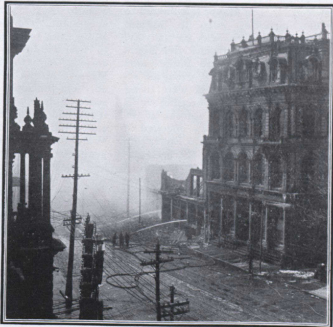
THE MINERVA BUILDING WHICH BARRED THE PROGRESS OF THE FIRE ON THE NORTH SIDE OF FRONT STREET, NEAR YONGE
