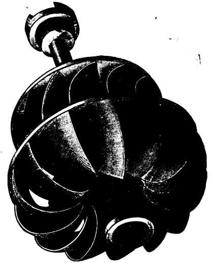
Cut Showing Wheel Removed from Case 84 per cent of power guaranteed
