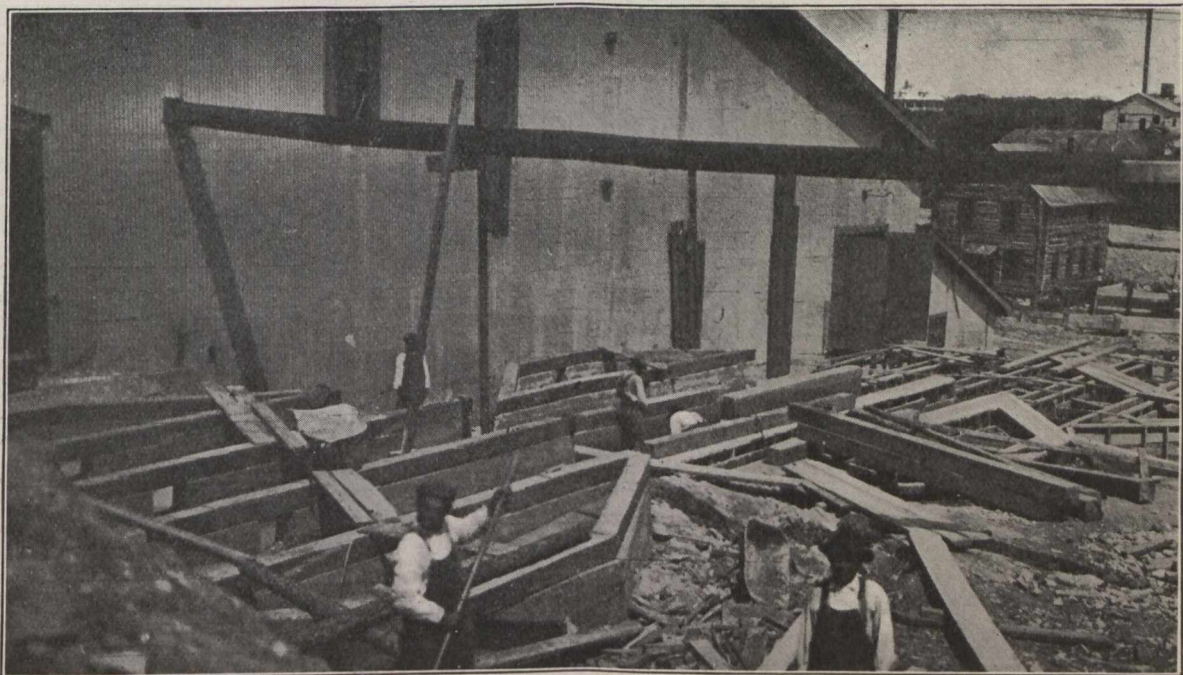
Constructing Foundations for Addition to McIntyre Plant
