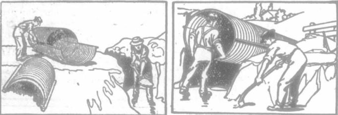
These pictures show how easily and quickly you can lay Pedlar Culvert. Comes nested, half-section within half-section—saving freight and cartage. Triple-thick Flat flange locking ribs on each side are clamped together by a simple tool—no bolts nor rivets needed. Joints are broken—only culvert you can do that with. Ends interlap. Will stand tremendous strains. Won't leak, nor buckle, nor crack from frost. Cheaper than wooden culverts.
