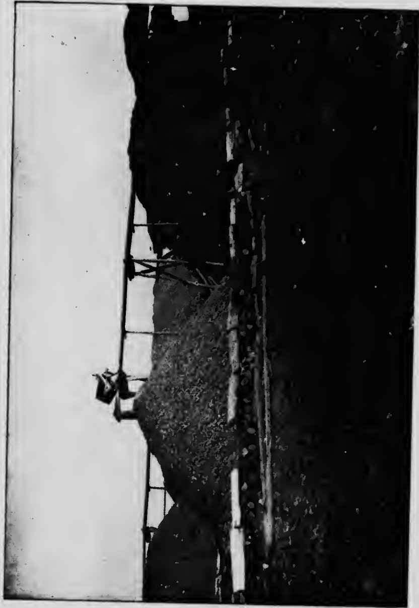
ROAST YARD AT COPPER CLIFF, ONT. Showing temporary trussle and general method of building roast heaps.
