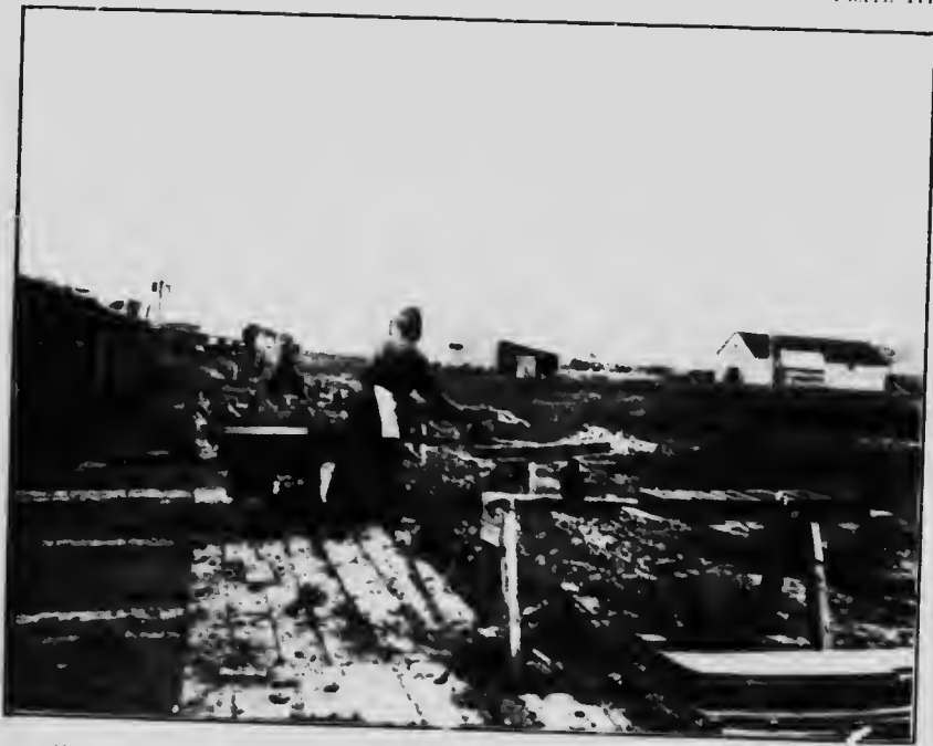
Conveyer and drying racks for soft mud bricks at Alsip's brickyard, Winnipeg, Man.
