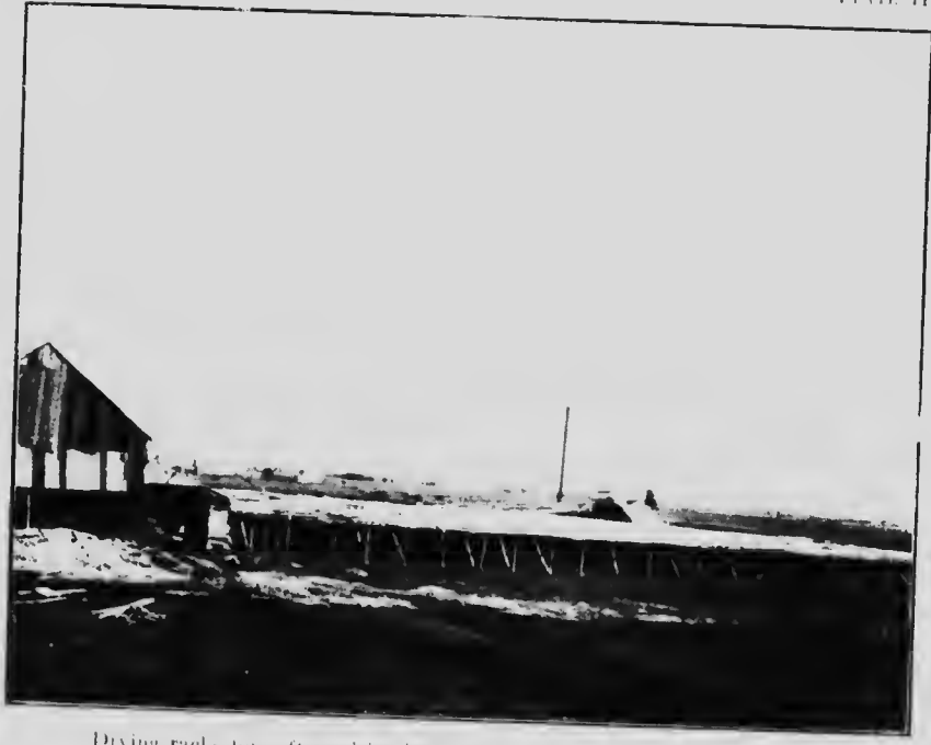
Drying racks for soft mud bricks, Cente City Brick Co., Winnipeg, Man.
