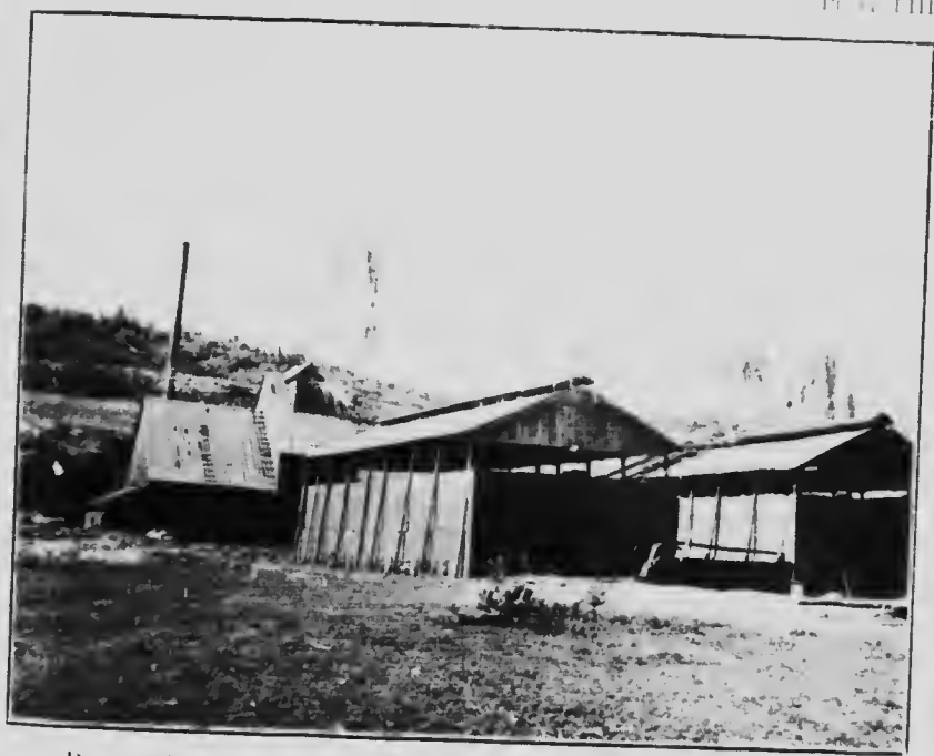
Dry-press brick plant at Blairmore, Alta., with bank of crinoid shales in rear
