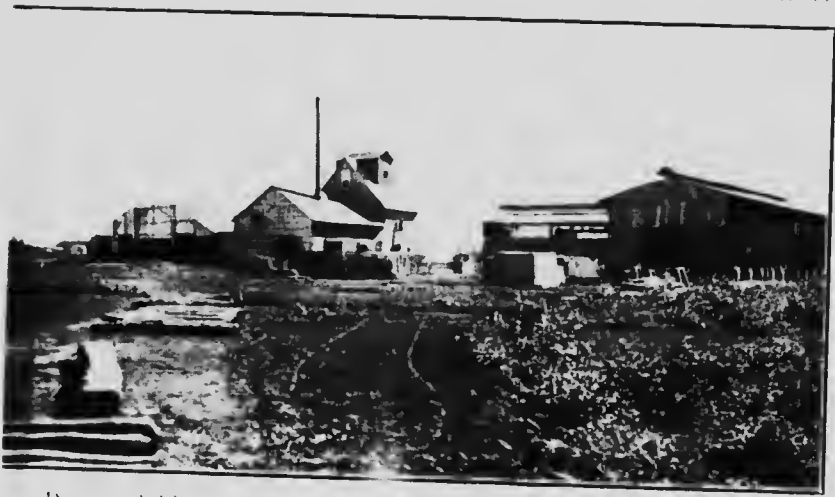
Dry press brick plant, using surface clay - Celtic Brick Co., Prince Albert, Sask.
