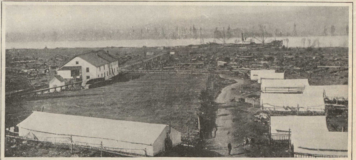
Clearing the Site of a New Ocean Port—The Pacific Terminus of the New Canadian Northern Line From Edmonton; Almost Opposite New Westminster, B.C. In This Picture the Clearing Camp is Shown. In the Background an Ocean Liner in Port Before the Site is Out of the Woods.
