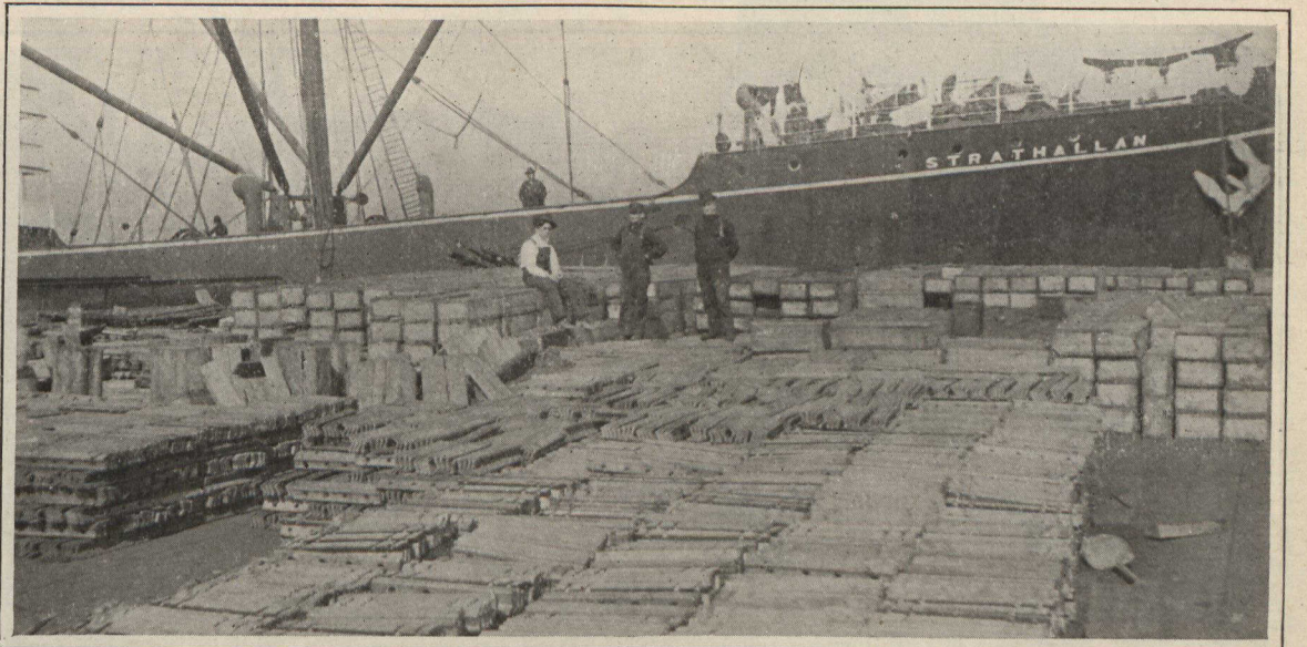
The Steel Rails and Fish-plates Shown in This Picture Came on Such Vessels as the Strathallan From Sydney, Nova Scotia, Down Around Cape Horn, and Up to Port Mann. The Water Haul of Eight Weeks Voyage is Cheaper Than the Land Haul—for the Extreme Western End of the Line.
