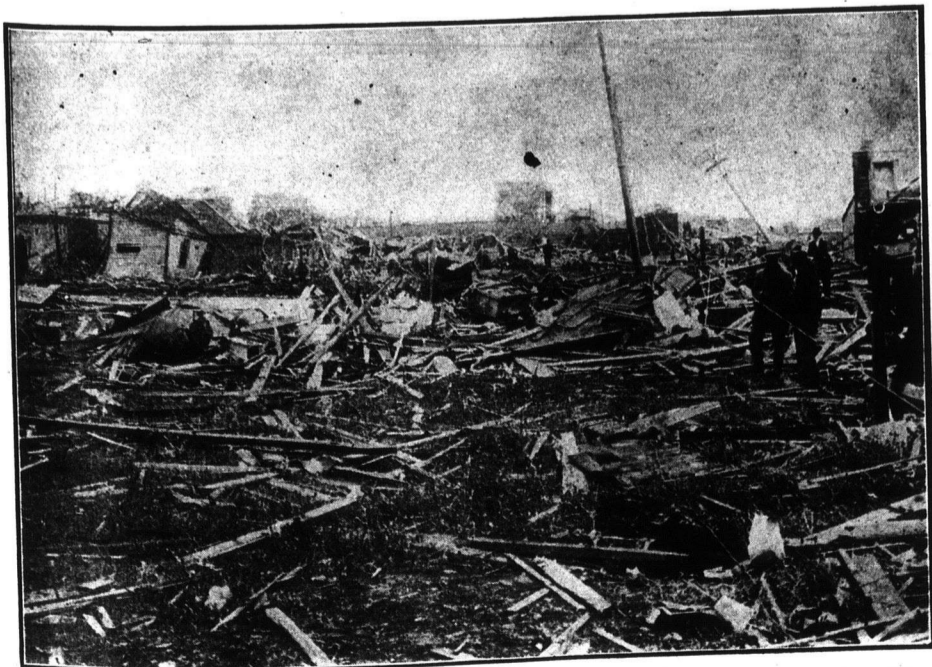
Showing a corner of a vacant lot covered with debris after the cyclone. This gives some idea of the way in which the timber was carried about.
