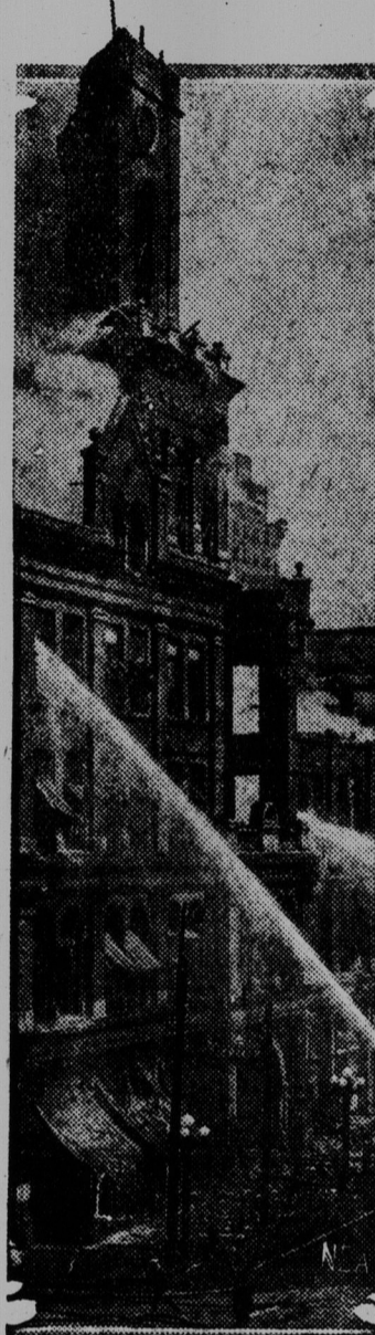
Several frames were injured and property damage of $1,000,000 was sustained when the city hall at Birmingham, Ala., was destroyed by fire. The public library, housed on the top floor, was a complete loss.
