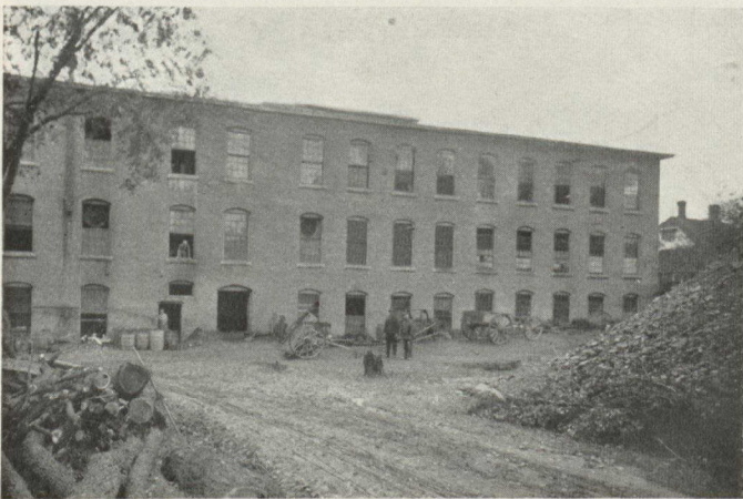
WEST WING AND SITE FOR NEW POWER HOUSE
