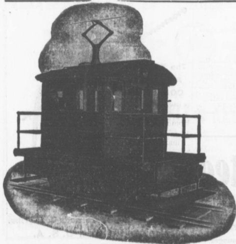
A TWENTY-FIVE TON ELECTRIC LOCOMOTIVE.
