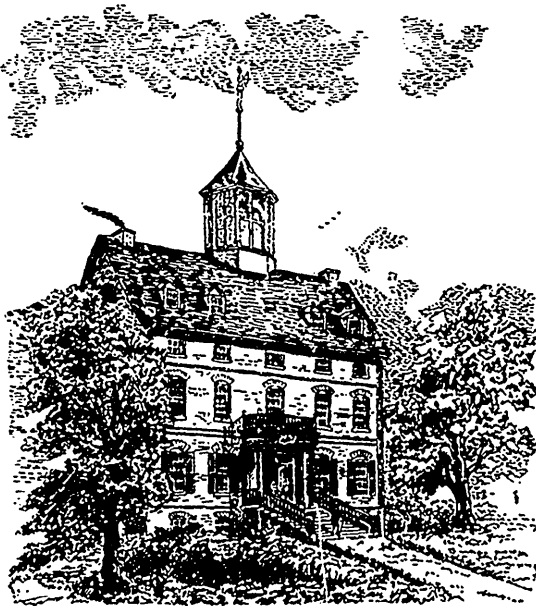
OLD PROVINCE HOUSE.
