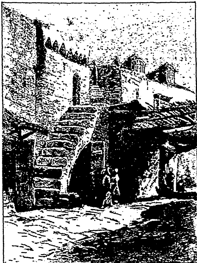
OUTSIDE STAIRWAY TO FLAT-ROOFED HOUSES.
