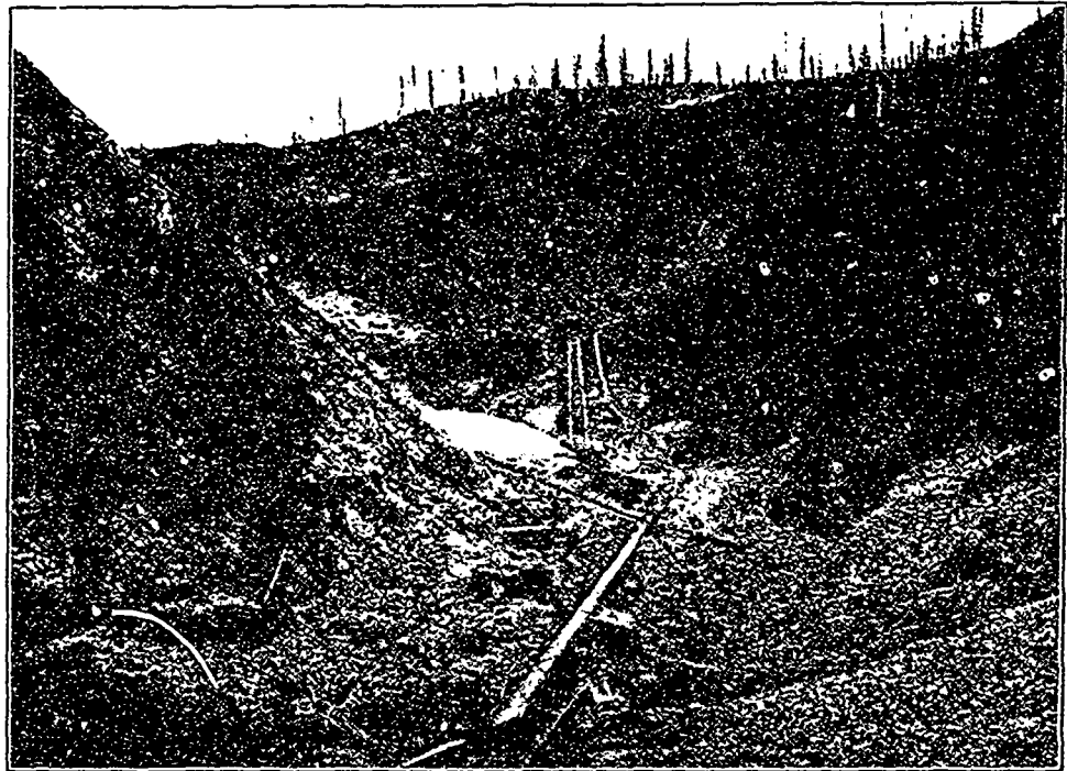
Pit No. I, Con. Cariboo Hydraulic Mine.—Piping Slope for Pipe Ladder to floor of workings on lower bench.
