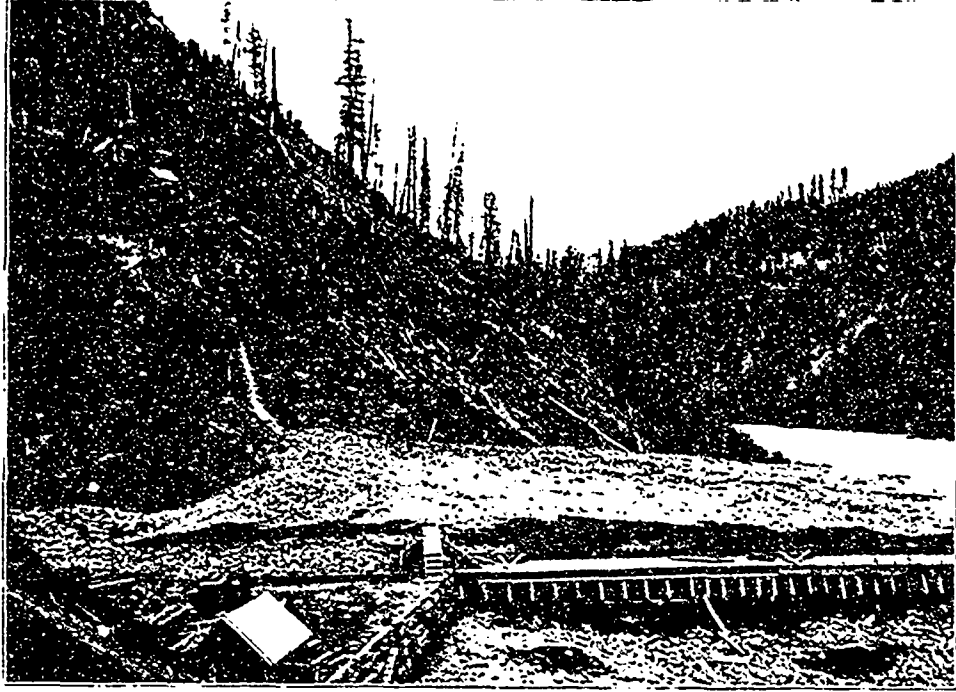
Con. Cariboo Mine Dumps into South Fork of Quesnelle River. Lower sluices 90 feet above high water. Upper system of sluices 150 feet above high water mark.
