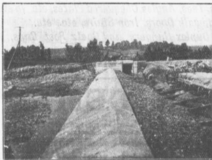
FIG. 1.—VIEW OF FACE OF R. FORBES DAM.
