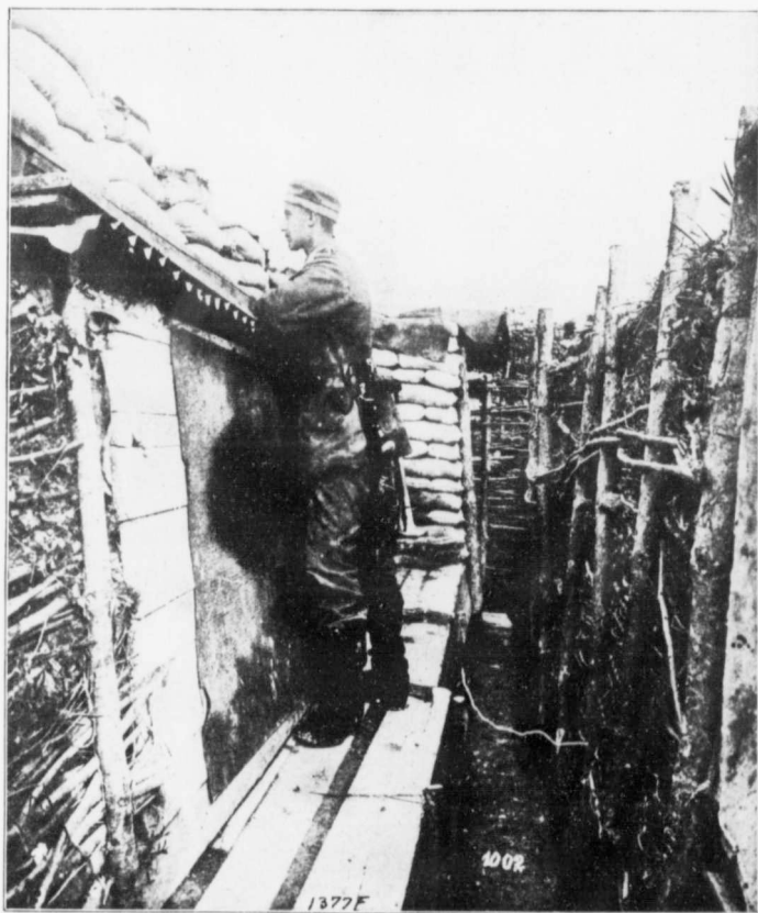
A German Lookout in a Waterproof Trench. A view of a sandbag-constructed trench on the German battlefront in the Western battle zone showing how carefully the trench has been water-proofed.
