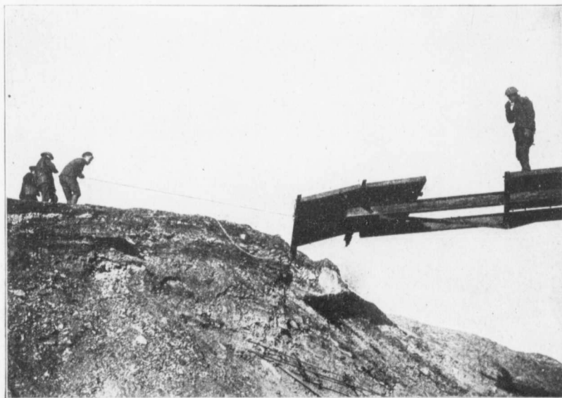
Canadians dismantling an old bridge on the Lens front.
