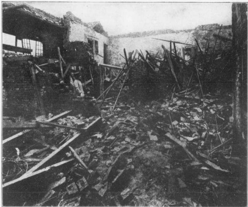
London air raid. Mother and son inspecting their home. They returned home from a visit and this mass of debris greeted their eyes.
