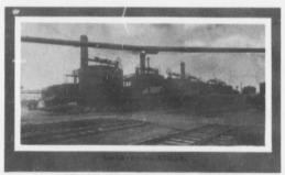
Oils are here freed of sulphur by copper oxide.
