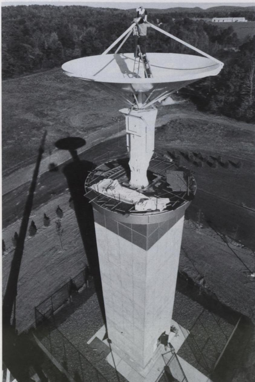
◀ Parabolic doppler radar antenna
