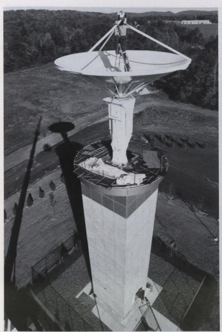
Parabolic doppler radar antenna
