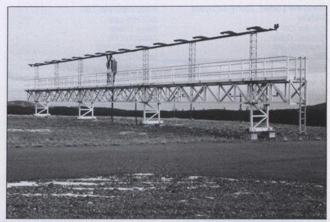
Instrument landing system (ILS) antenna support structure
