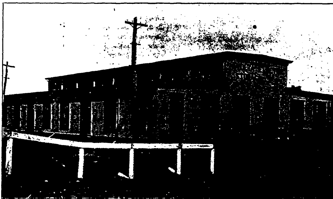
WORKS OF THE VOLTA ELECTRIC STORAGE CO., HAMILTON, ONT.
