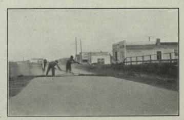
Experimental pavement at Edmonton, laid under direction of S. V. Ells, of the Mines Branch, to demonstrate use of Alberta's bituminous sand deposits.
