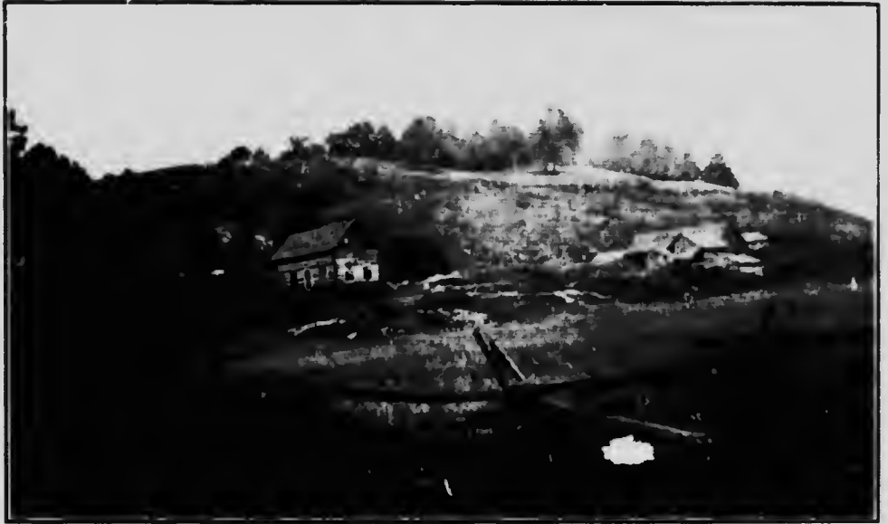
TYPICAL UPLAND FARM AND FARM BUILDINGS
