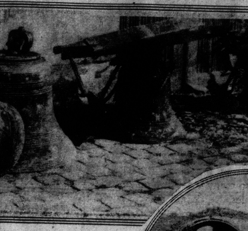
All that remained of the chimes after the German guns had demolished the cathedral.
