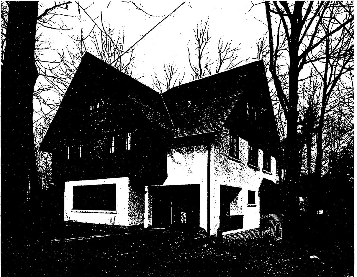
Residence of Geo. Howell, Toronto, Ontario—Eden Smith & Son, Architects.
