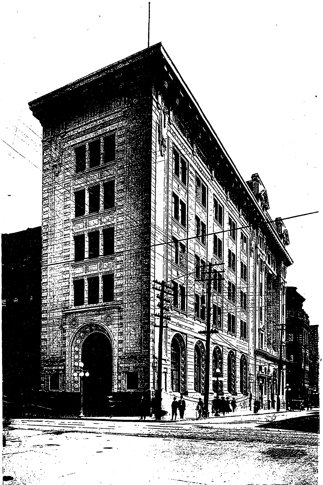
Union Bank of Canada, Toronto, Ontario. Darling & Pearson, Architects.
