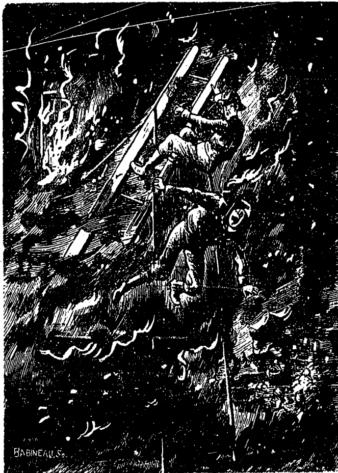
Two of our gallant firemen, T. H. Hogan and Wm. Stewart, of No. 3 station, jumping from a ladder in consequence of the fall of Kirkpatrick's cooerage, corner of Prince and Ottawa streets falling in on Thursday morning. They had a miraculous escape from death only having received a few injuries.
