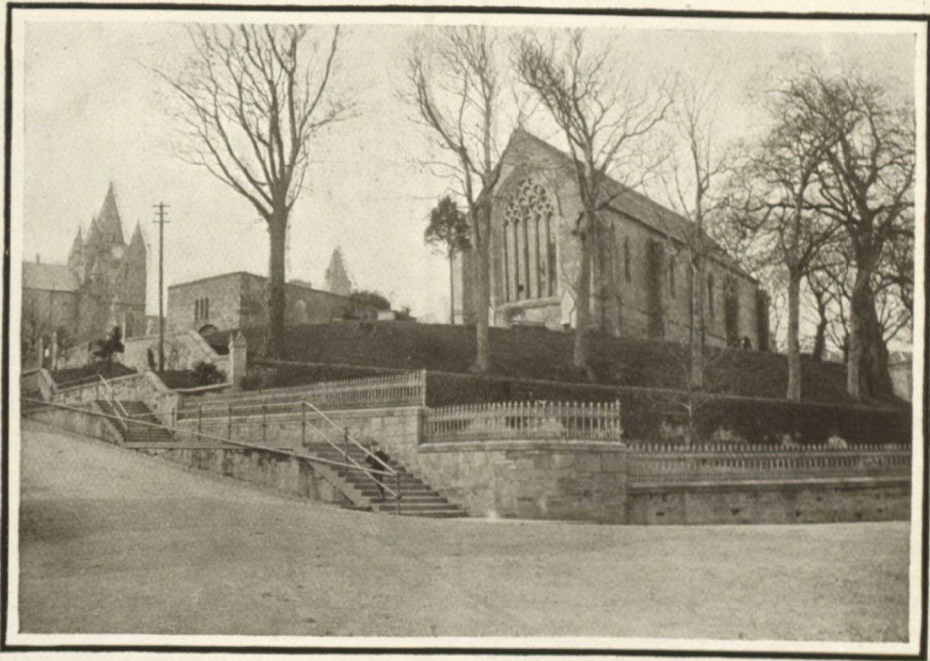
THE OLD COLLEGIATE KIRK OF ST. DUTHIE, TAIN, SCOTLAND It was built in 1370, and to the left stands the Chapter House, roofless
