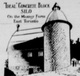
Erected at Dentonia Park Farm for Mrs. E. D. Massey. 34 feet high—15 feet diameter—capacity 180 tons. Built of "Ideal" Blocks.
