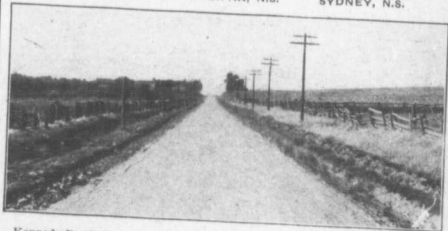
Kennedy Road, Scarborough Township, York County Highway Board, Ontario. Constructed with "Tarvia-X" in 1916.
