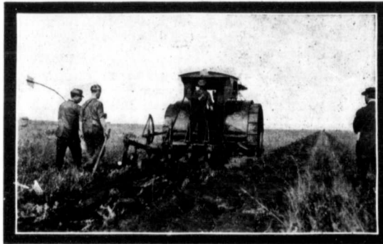
The I.H.C. Tackling a Rough Job
