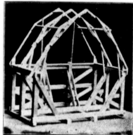
Frame Work of Plank Frame Barn
