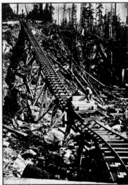
Incline Tramway to dam and Trout Lake portal of tunnel.
