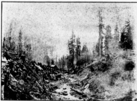
Trout Creek Dam Site in process of clearing.
