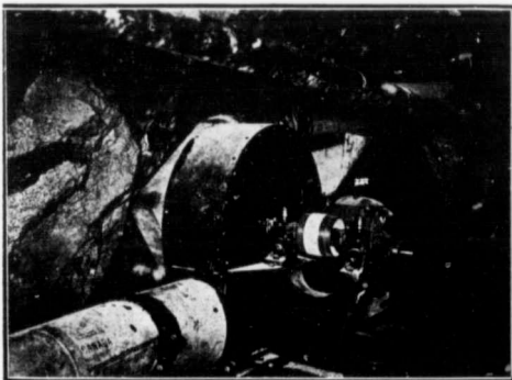
Ventilating station at Coquitlam Heading.
