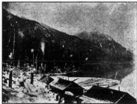
Coquitlam tunnel camp and plant.
