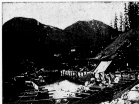
Sluicing out excavation for concrete dam.
