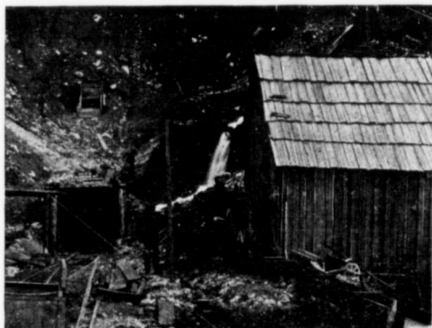
Trout Lake Portal, sluicing out the Portal Excavation.
