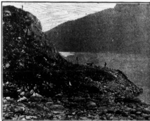
Excavation at power house site.
