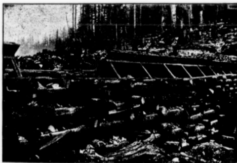
Temporary log crib dam in Trout Creek, to control the water during construction of the concrete dam.
