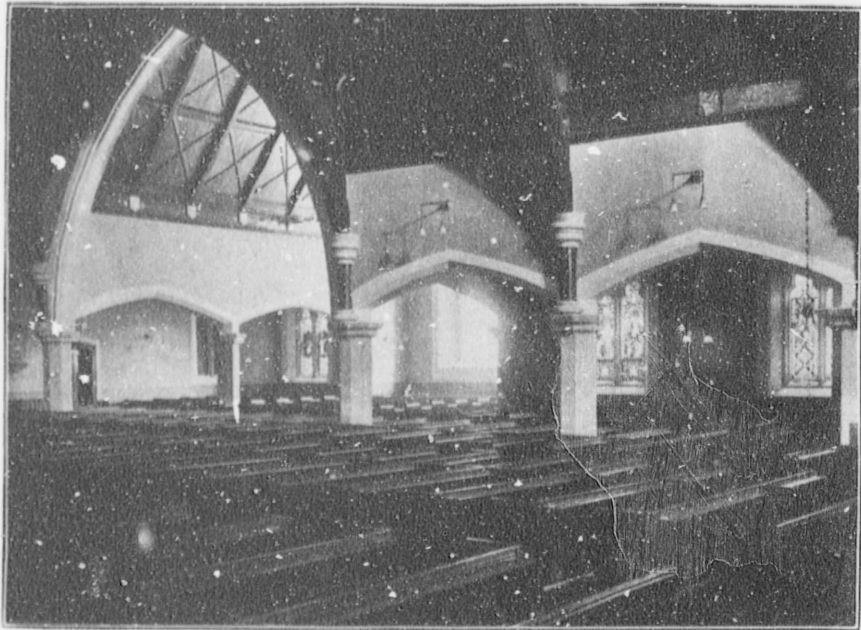
INTERIOR OF NEW TRANSEPT AND WING, 1914.
